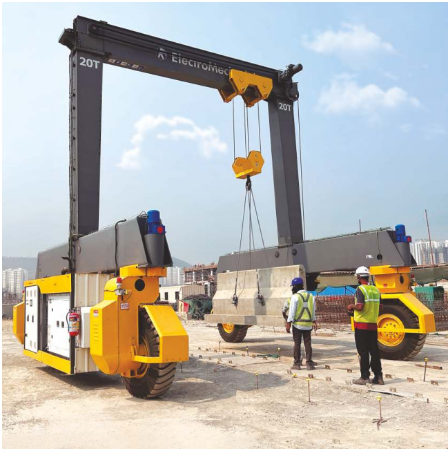
Handling of precast segments at a casting yard
