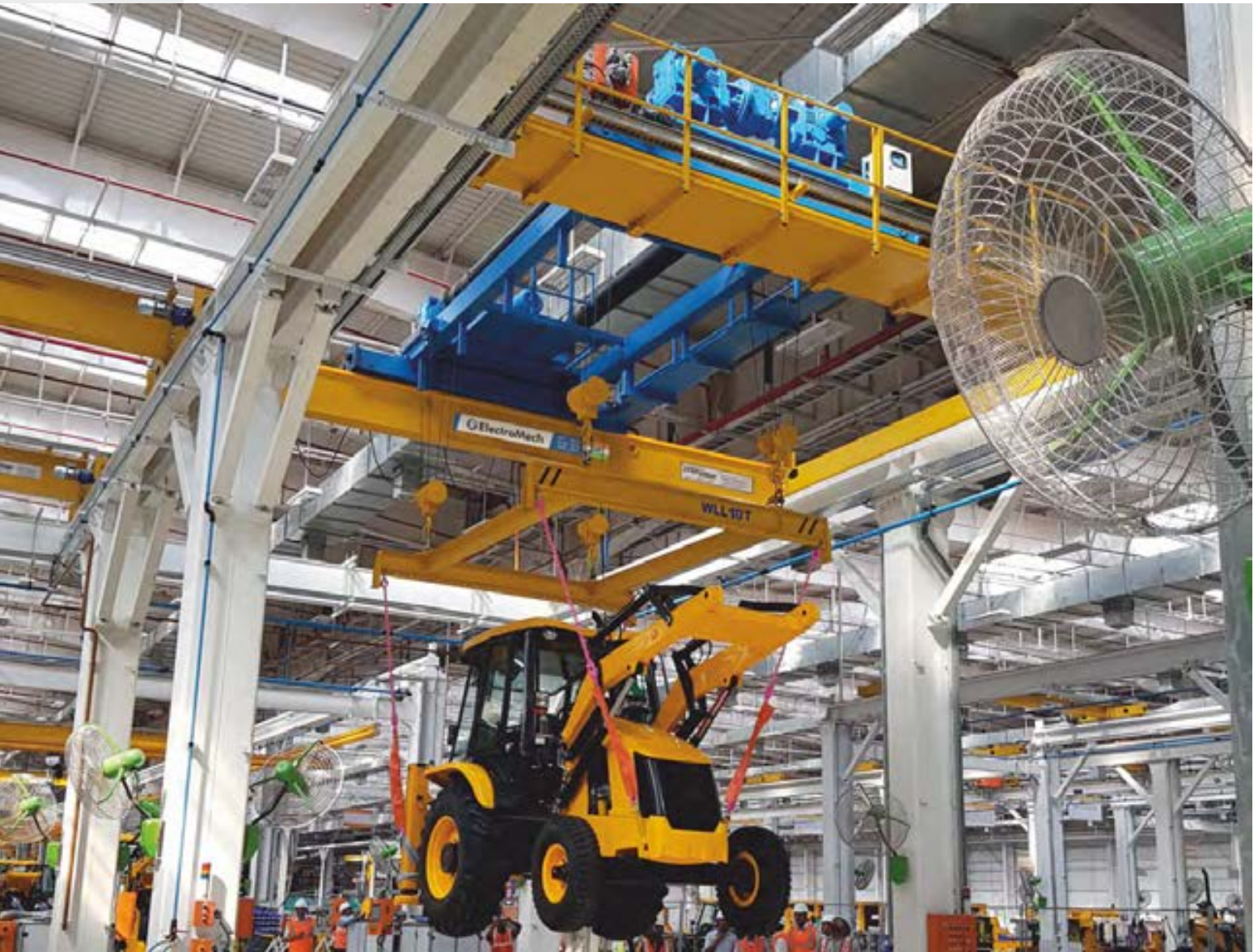
Customised double girder crane on vehicle assembly line
