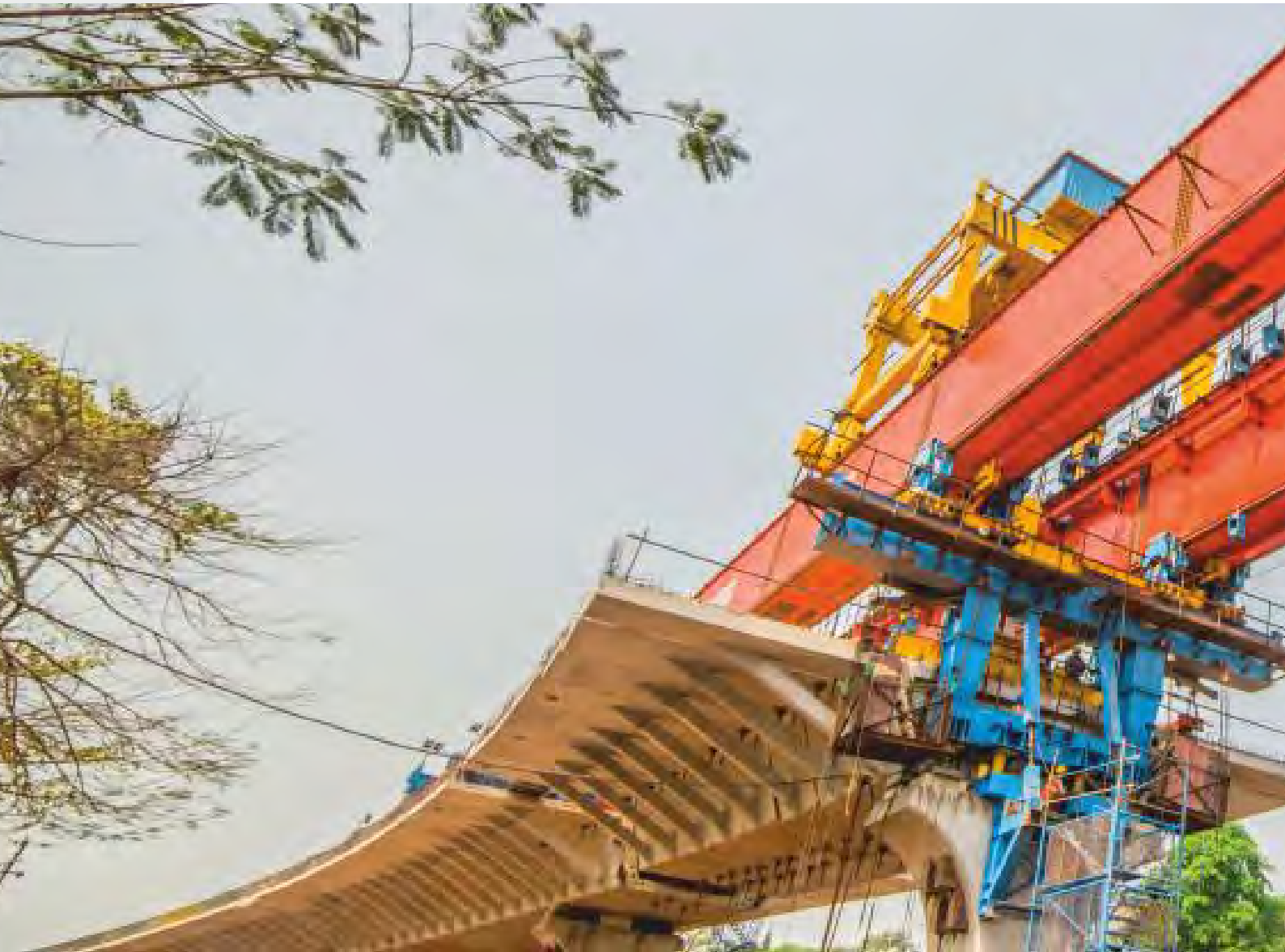
150t gantry crane for launching girder
