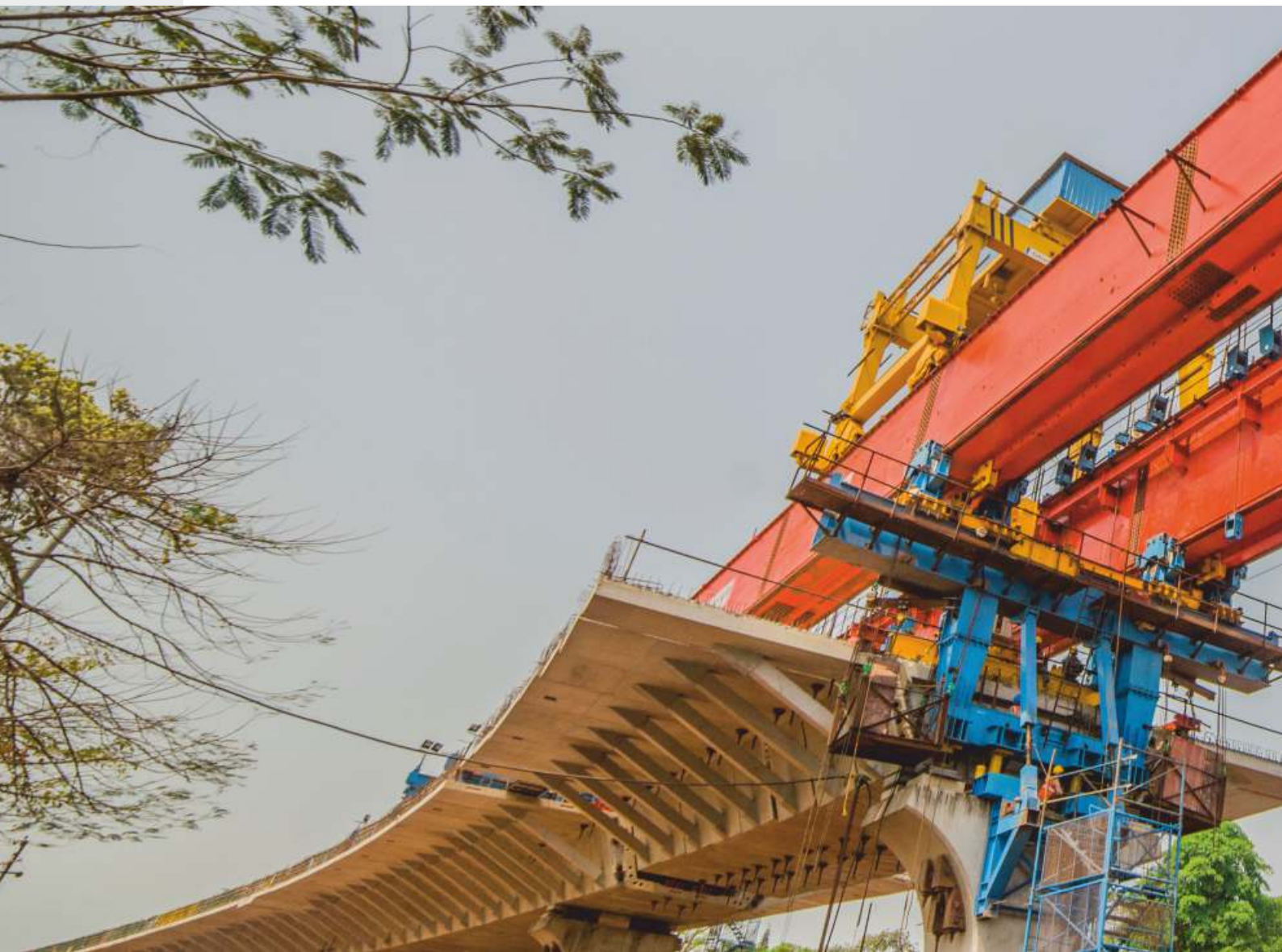
150t gantry crane for launching girder
