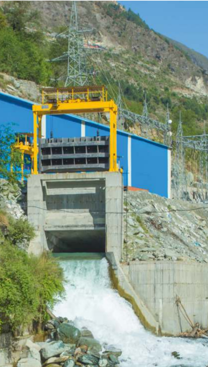
Double girder gantry crane for operating sluice gates installed on a dam in the Himalayas
