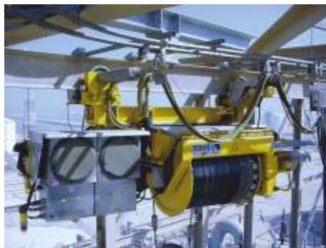
Arduous working conditions in Qatar: dust, sand, heat and saline atmosphere have no adverse effect on the wire rope hoist.
